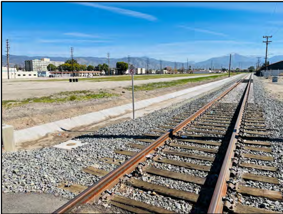
Plate 6.1-4: Overview of the subject property from the southwest property corner, facing northeast. The cleared and graded surface of the property are visible.
